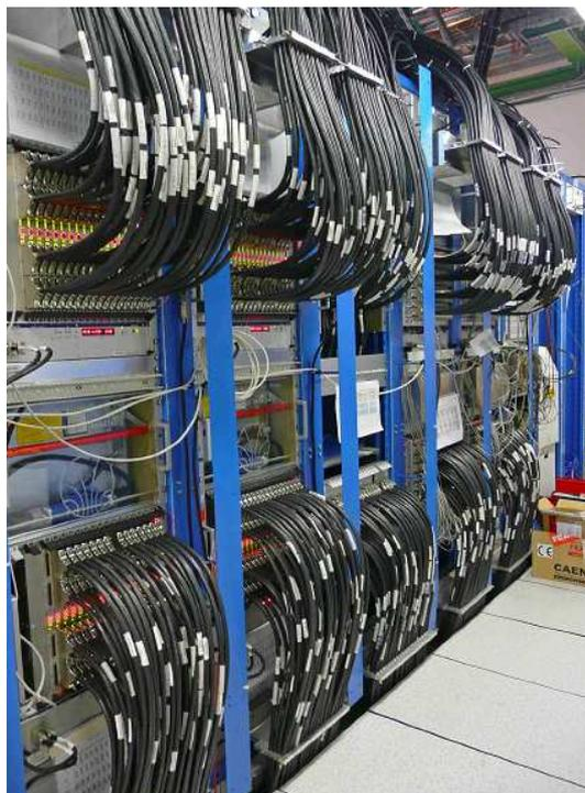
**Figure 6.** Short analogue cables for  $\eta > 0$ , from Receivers (two racks at right) to PPMs (two racks at left).
