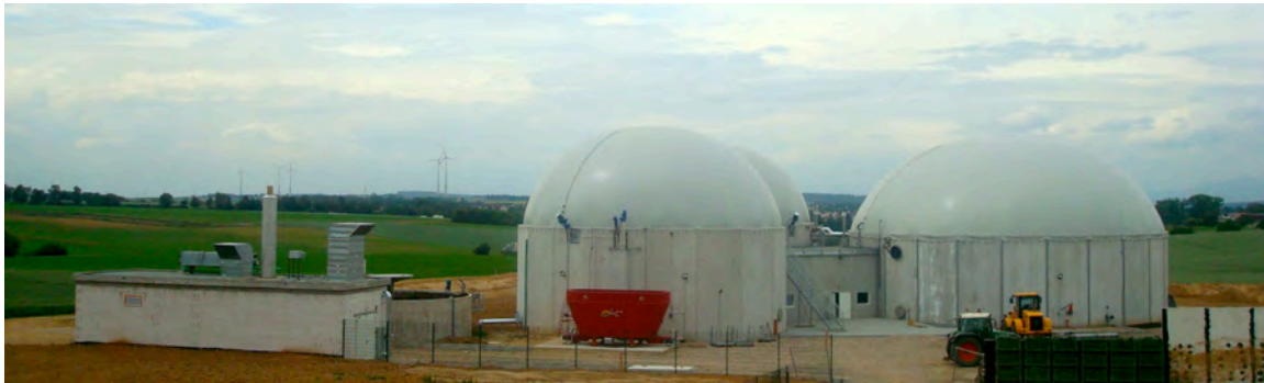
An example for a 1 MW anaerobic digester power plant fed with corn as well as animal excrements.
