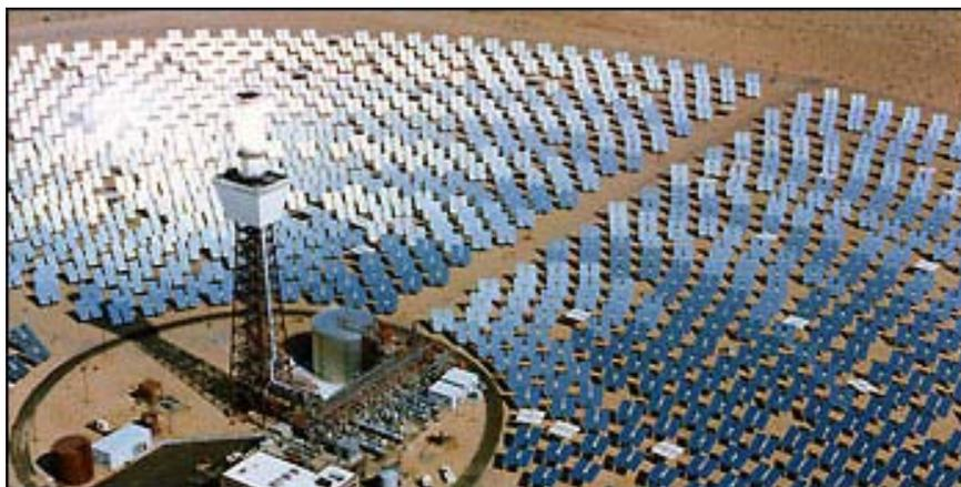
**Figure 4-7. Aerial View: Solar Two, 10 MW Thermal Tower Plant with Mirrors**
