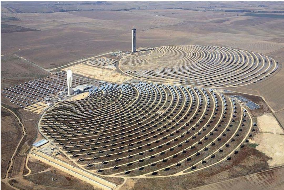
**Figure 4-9. Aerial View: Solar Thermal Power Towers with Heliostat Mirrors**
