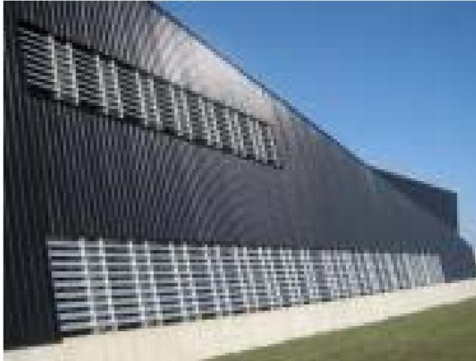
**Figure 5-5. Solar Ventilation Air Heating Installation**
