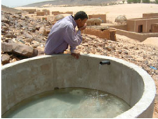
EWB-USA project— Lemraiveq, Mauritania : water well development
