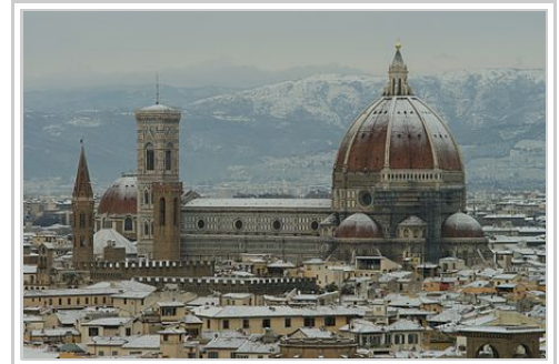
The Santa Maria del Fiore cathedral in Florence, which has the biggest brick dome in the world, [40][41] and is considered a masterpiece of Italian architecture and world architecture.
