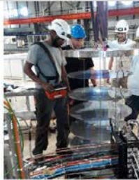
Manhole plug installation
