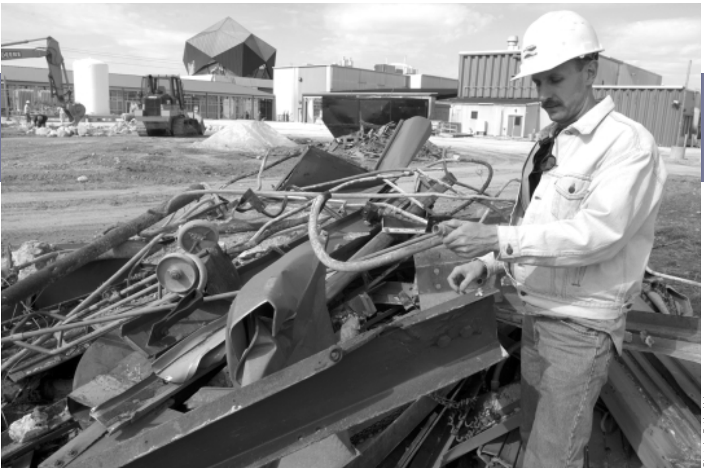
Eric Mieland of Fermilab's Environment, Safety and Health section examines material that has been removed from the "deconstruction" of the old Neon Compressor Building in the fixed-target area. New construction methods mean that nearly 85 percent of the material from old buildings in this area will be recycled, reducing costs and enabling a more complete cleanup. Mieland calls it a "paradigm shift" in the way old buildings are removed at the end of their useful life.
